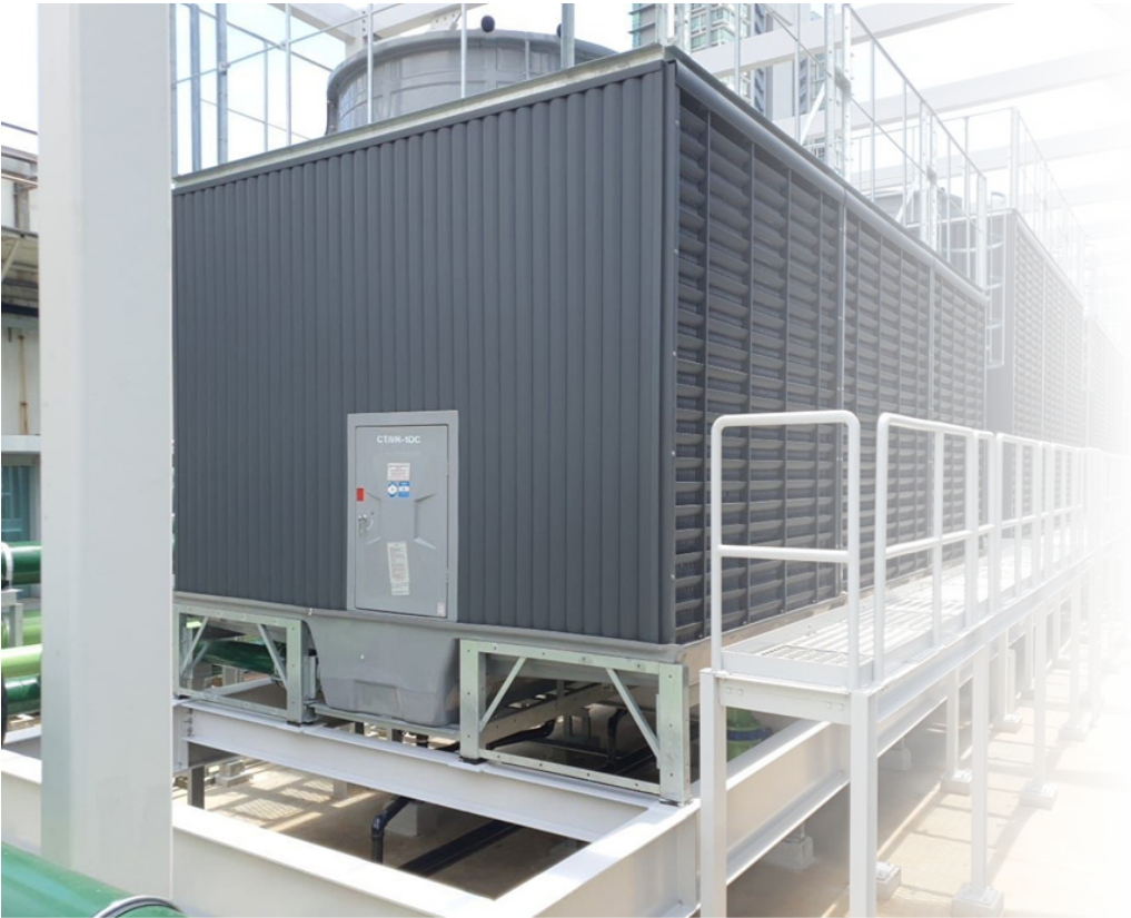
▲ The new cooling tower for the chillers
