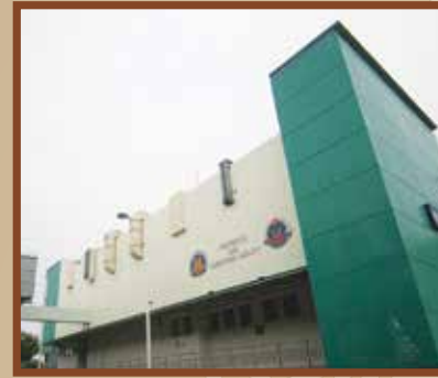
Protective & Analytical Facility (PAF) at Tuas Checkpoint
